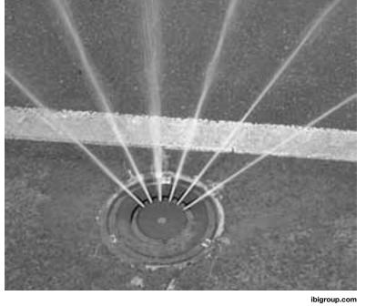
The FAST system automatically sprays an anti-icing liquid onto problematic stretches of roadway, such as bridge decks.
