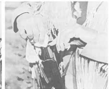
4. Trim excess patch with a sharp knife.
