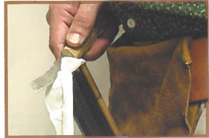
4. Trim excess patch with a sharp knife.
