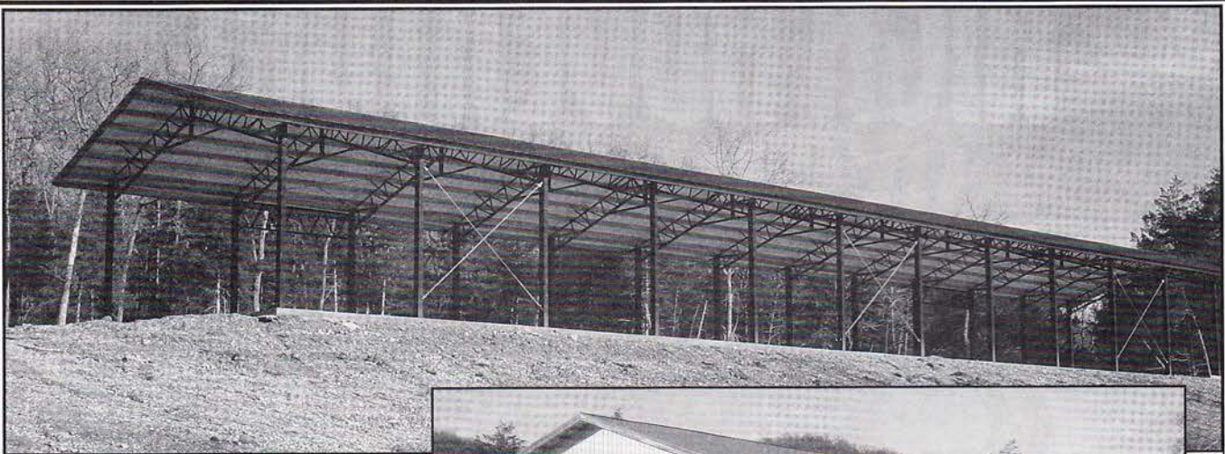
Pictured above: Two covered shooting pavilions (24'x120' each).
