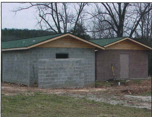
Example of a new and renovated shower house
