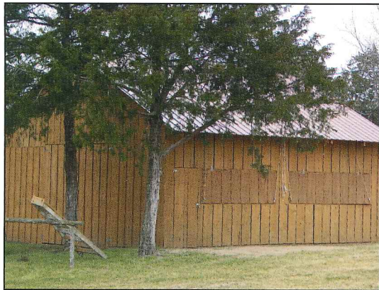
Renovated exterior of Blacksmith Shop
