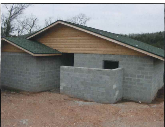
Closeup of a new and renovated shower house
