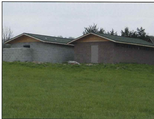
Example of new and renovated shower house
