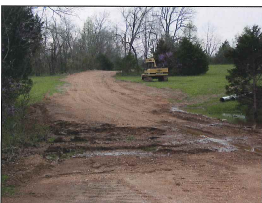
Site development on roads
