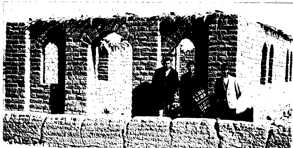
This new church with adobe walls is ready for the roof. These Bolivian brethren will conduct services here soon.
