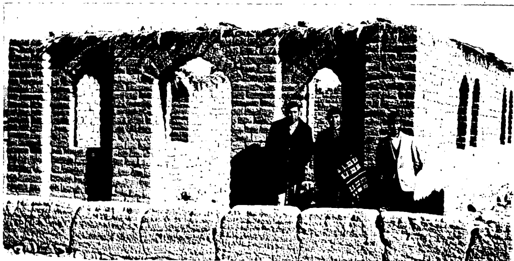
This new church with adobe walls is ready for the roof. These Bolivian brethren will conduct services here soon.
