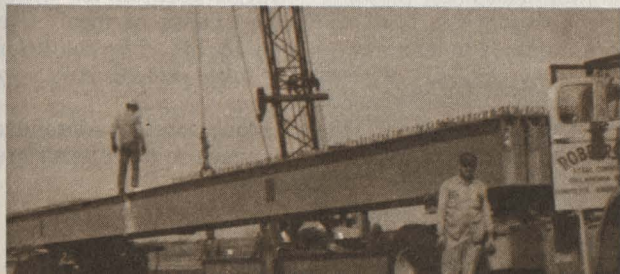
Jimmy R. Milligan drives truck delivering steel beams.
