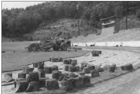
In 1970, the natural grass playing field was removed from Conrad Stadium and replaced with an artificial surface, the first in the Carolinas.
